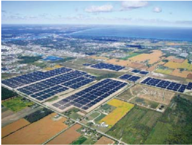
Figure 7.7 Sarnia PV power plant, Ontario, Canada, 97 MW peak, 1.3 million modules (photo courtesy of First Solar) [13]
