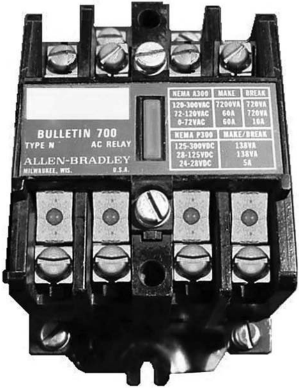
FIGURE 7-11 Allen-Bradley control relay
