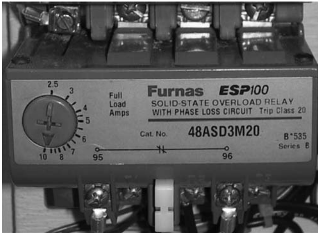
FIGURE 8-9 Furnas electronic overload unit
